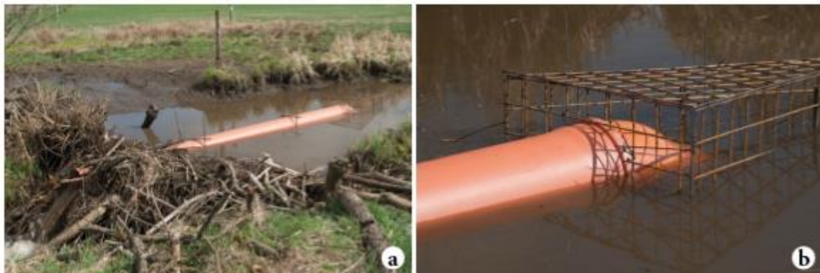
Figure 29: Drainage of a beaver dam: into a dam inserted pipe with a knee in an inflow and with a protective cage (a); detailed inflow of the pipe and protective cage (b), Czech University of Life Sciences Prague, 2016
